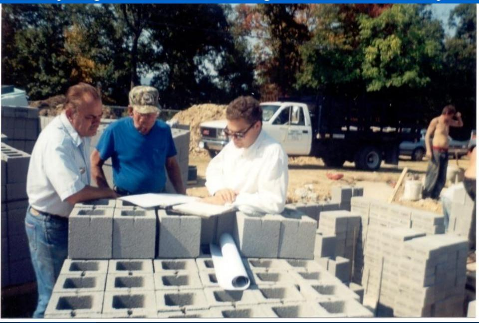
Form for isostatic pier for telescope, eventually contained 33,000 lbs concrete and has its own separate foundation from rest of building
